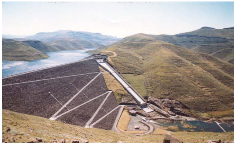
The majestic zig-zag rockfill concrete face Mohale dam. Transferring 9.2 cubic metres of water into Katse dam some 32km away.
